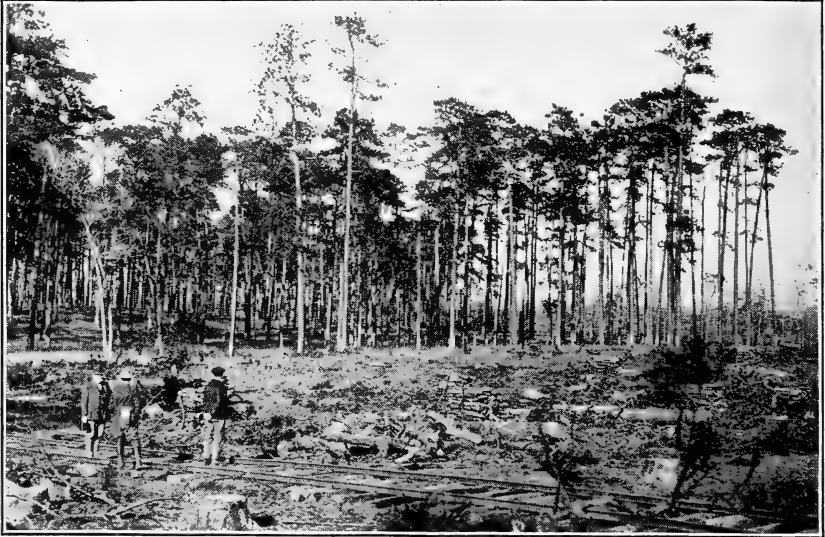
FIG. 1.—Here is going on the complete removal of the forest cover, and it is not likely to return naturally. After being cupped for two years, practically every pine is cut for saw timber or pulpwood. The tops and culls are being worked up into pulpwood; but, regrettably, all the small young trees down to 4 inches are being taken. This type of logging, with the exception of the close utilization, is widely practiced over the longleaf belt
